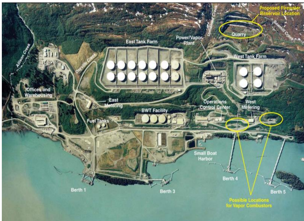
Fig 5. Aerial-view of VMT Alaska BWT facility (Source; Alyeska Pipeline service)
