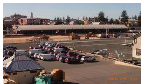
Photo. 8 Wharf and station
