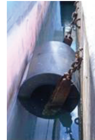
Photo. 11 Fender of wharf
