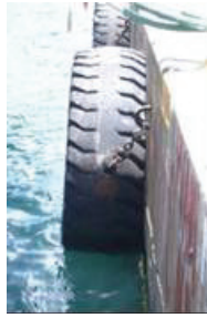
Photo. 10 Fender of wharf
