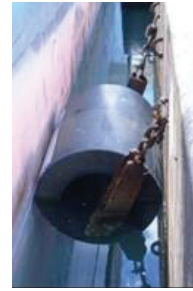
Photo. 11 Fender of wharf
