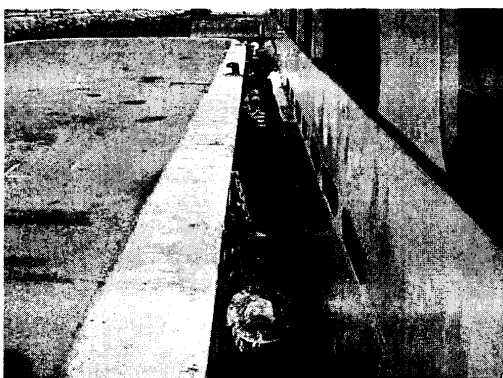
Photo 6. Fender of the berth.
