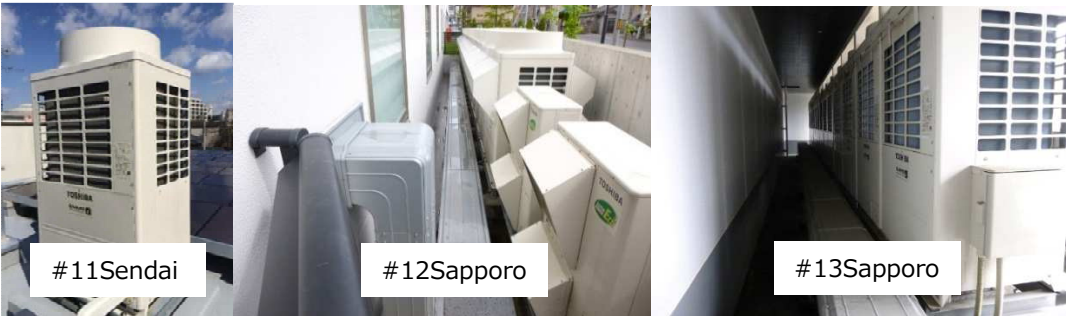
Figure 4.9-5 Installation conditions in Sendai and Sapporo
