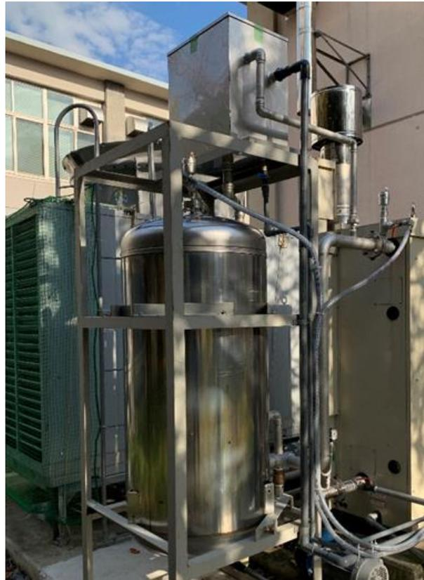
Fig.16 Temperature Adjusting Tank and Expansion Tank
